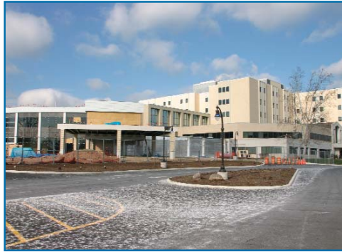
As LMH celebrates its 109th birthday, construction is underway for the Critical Care Pavilion which is expected to open in late 2007.
